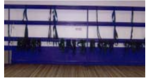
Right Side Wall Pipes
