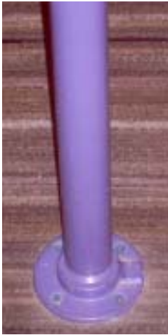
^Pipes bolted into the floor
