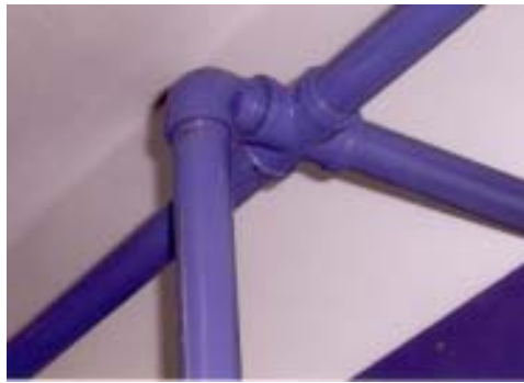
^Close-up of center fittings.
